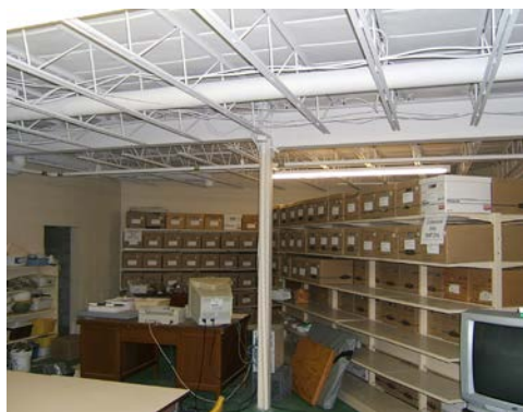
The collections area with the new insulation and drywall and the ceiling painted.
